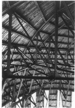
17e. Church Am Steinhof, structure between domes.
