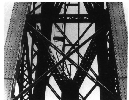
5b. Viaduct at Garabit (1880-84), Gustave Eiffel, detail.
